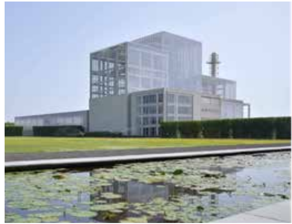
Figure 11: Waste-to-Energy Plant, Jamnagar
